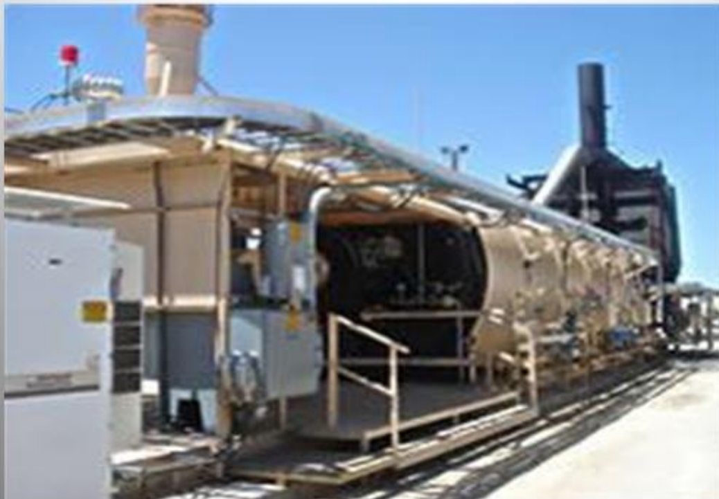
APIN™ EORSG located at East Texas oilfield
