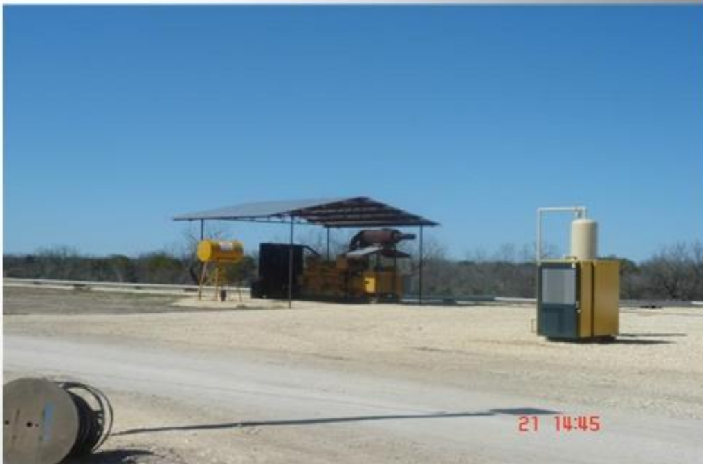
APIN UPS System for APIN EORSG support.
